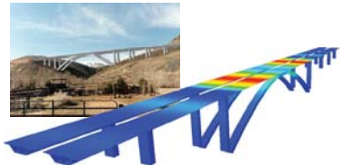
Galena Creek Bridge (Nevada, USA)
