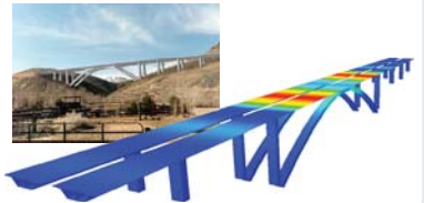
Galena Creek Bridge (Nevada, USA)
